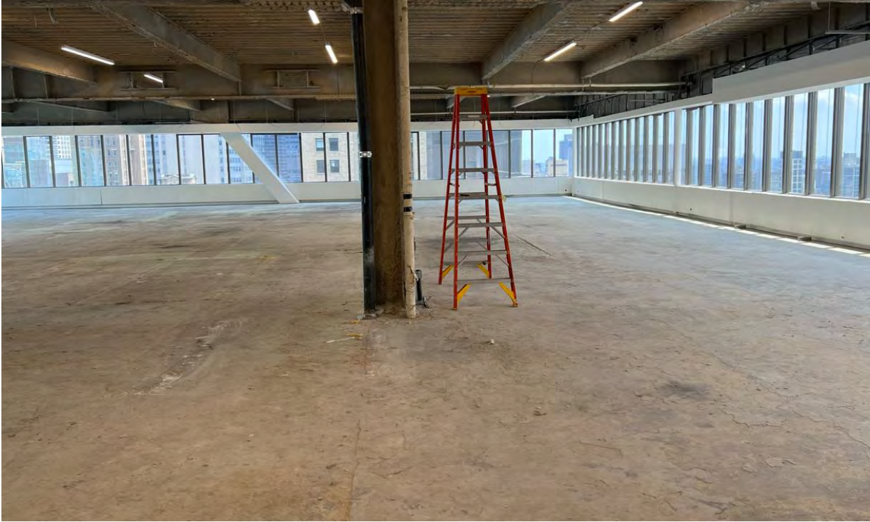
View of the Subject Vacant Office Space
